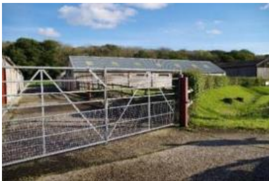
Looking East from entrance
